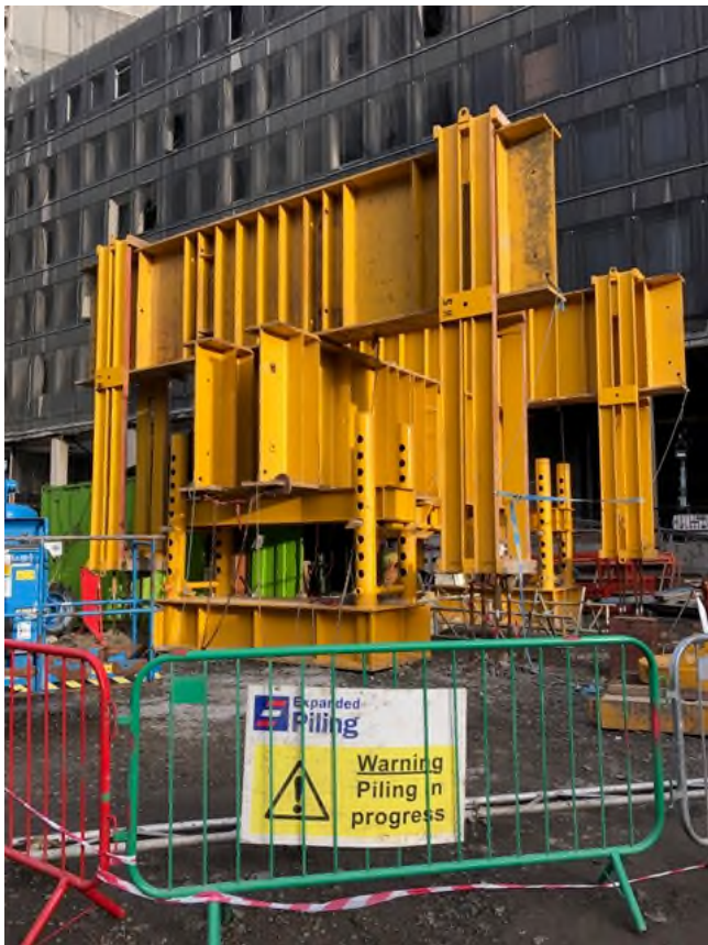
Figure 5 - 14MN Pile Test Frame
