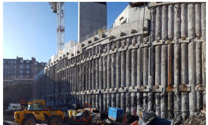
Figure 3 – View on wall anchors along James Craig Walk
