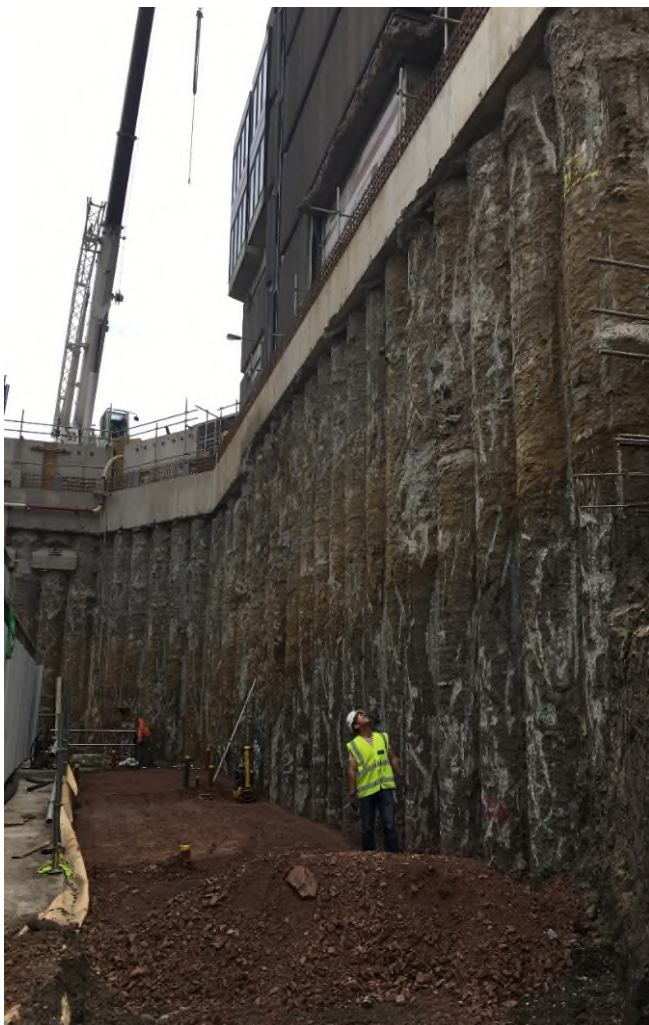
Figure 6 - 12m high free-standing cantilever wall
